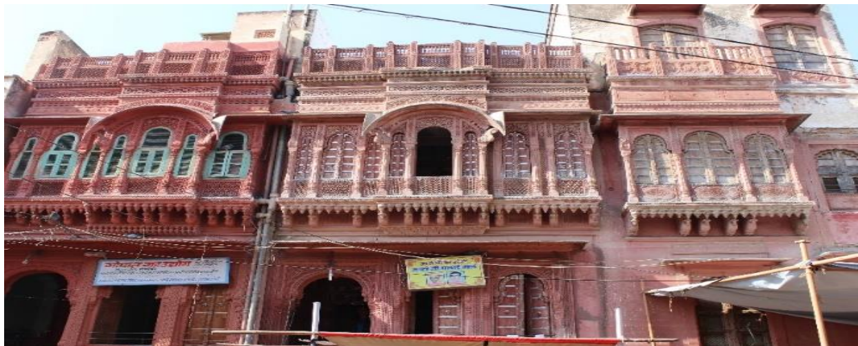
Fig. 3.2 Front Facade of the Haveli
