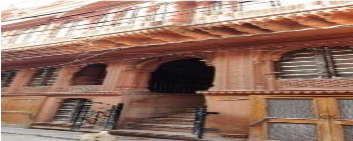
Fig. 5.3 Overhanging first floor of the Haveli
