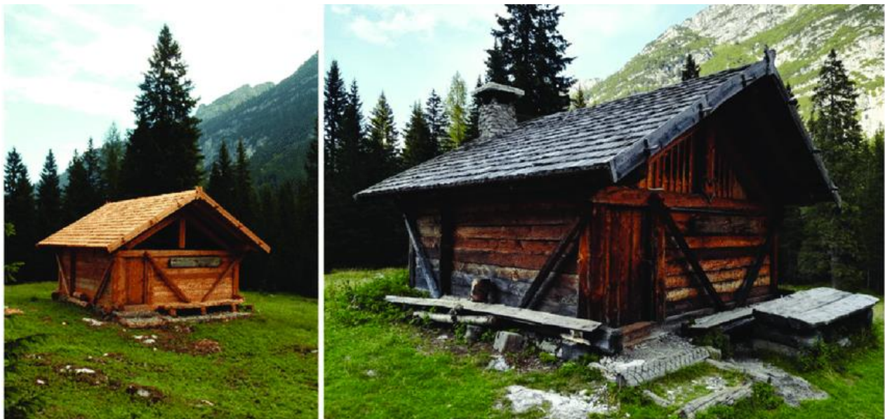
Fig. 2.6 Traditional Wooden House [19]
